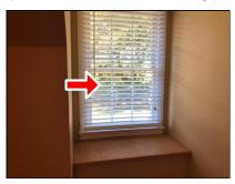
(2) Evidence of water intrusion was noted in between the panes of windows in the first floor middle front room and at the front entryway. This indicates a blown seal. Recommend repair.
