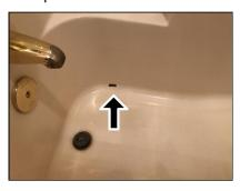
(4) Diverter valve in the first floor right rear bathroom did not seal completely while operating the shower head. Recommend repair.
